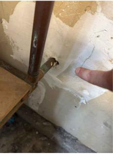
7.3.2 Hot Water Source **DEFECT AT TPR VALVE DISCHARGE**
